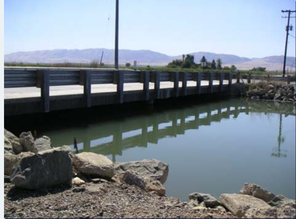
Fairview Road Bridge
